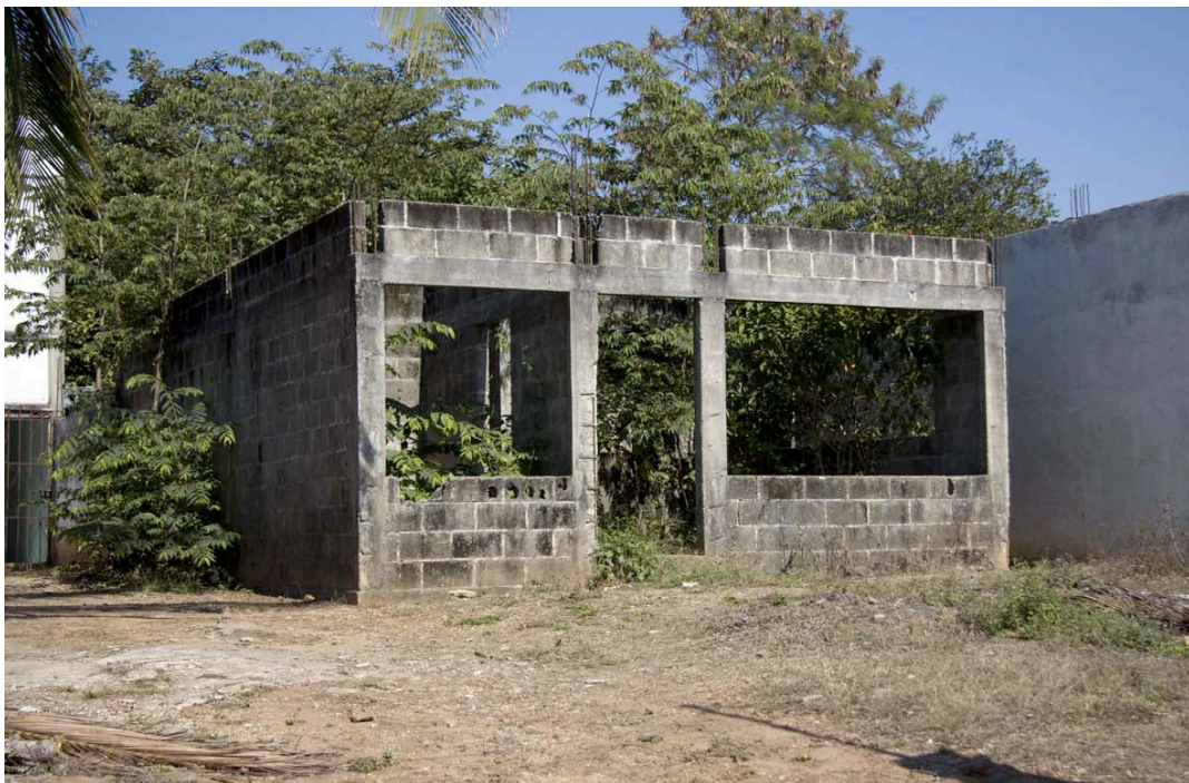
A home in construction – temporarily abandoned Tres Valles, Veracruz, Mexico
